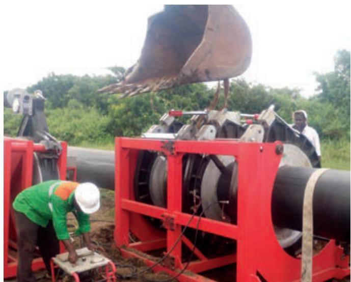
Polyethylene pipe butt welding
